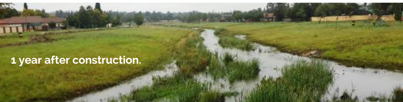
Early in-stream re-establishment to mitigate post construction erosion risk.
