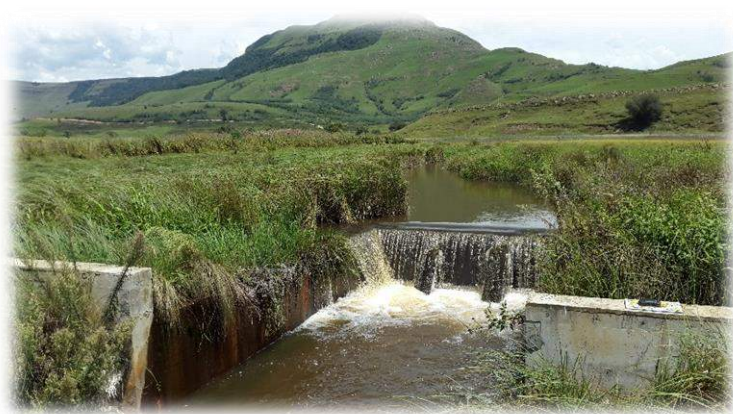
Figure 26 Concrete weir plug within a drain in the Hlatikhulu wetland in KwaZulu-Natal 89 .
