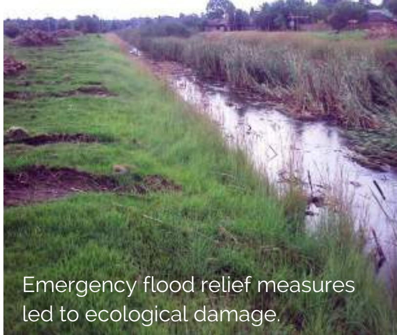
Reed infestation in canalised drain reduces hydraulic capacity.
