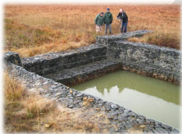
Figure 27 Gabion weir plug within a drain, Golden Gate National Park, Free State 90 .
