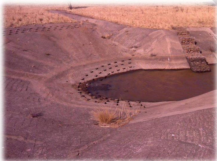
Figure 25 Hyson-cell geo-chute with concrete baffles for headcut stabilisation in a seep, Free State 88 .
