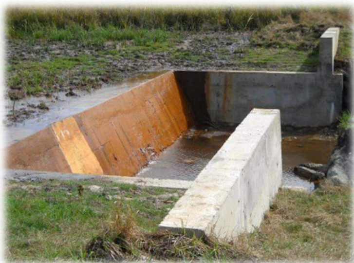
Figure 24 Concrete drop inlet weir for headcut stabilisation 87 .
